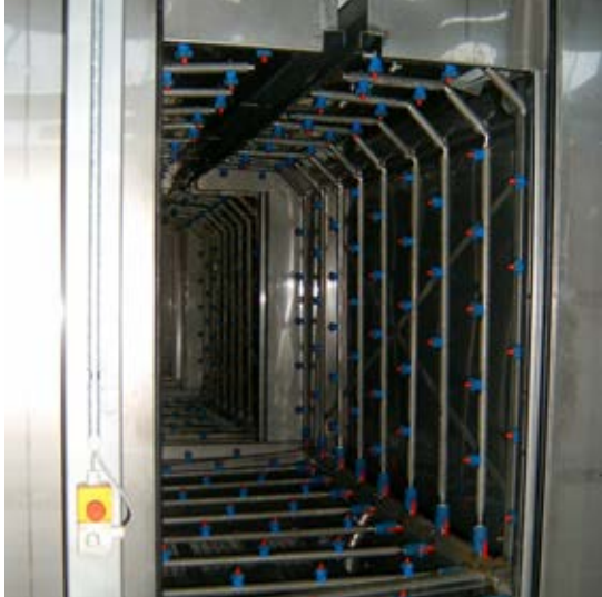
Figure 27: Unit for chemical pre-treatment
